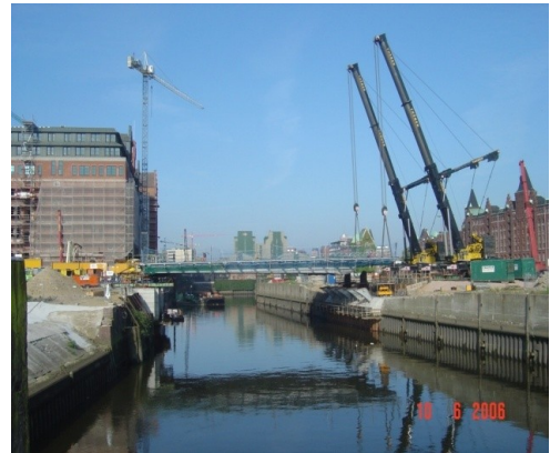
Brooktorhafen bridge during move
