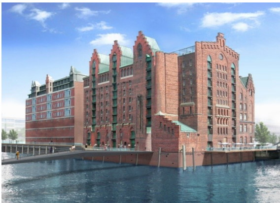
New museum bridge to the quai storehouse B
