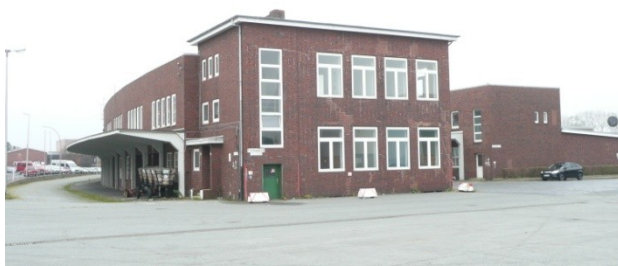
Fish processing factories before start of construction
